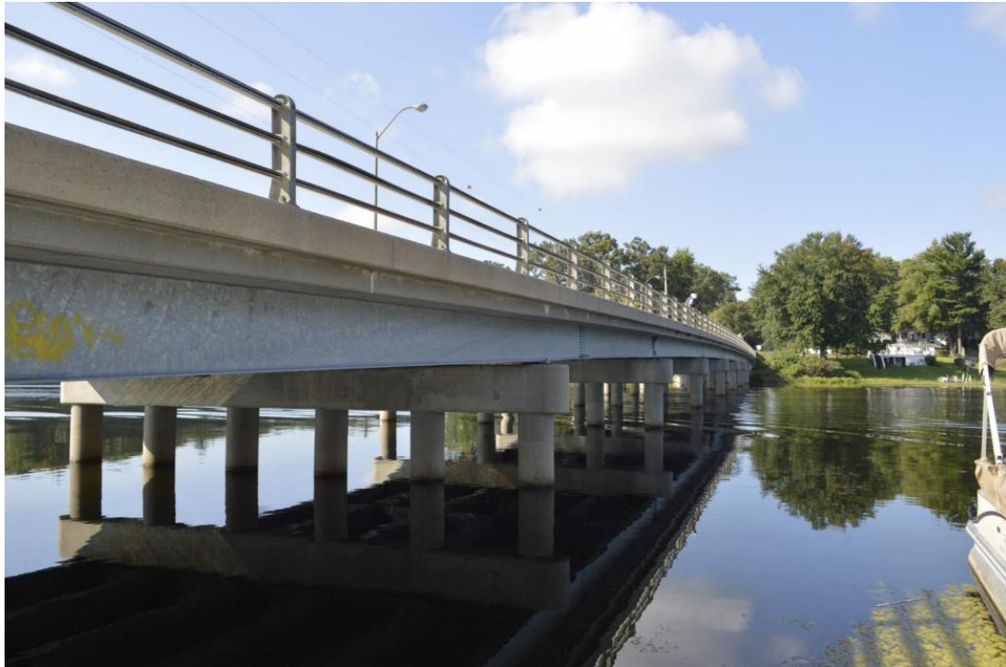
Obr. 1 - Stearns Bayou Bridge v Ottawa County, Michigan (zdroj AGA)
